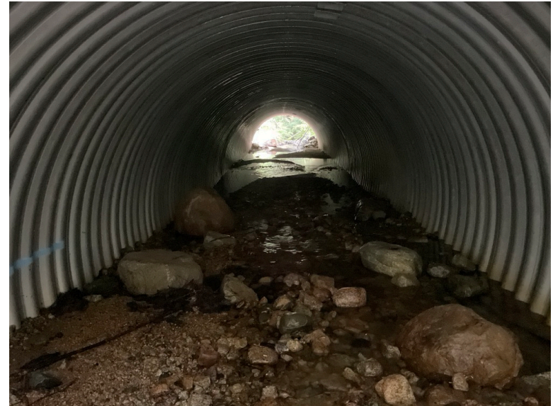
Looking Downstream Through CMP
